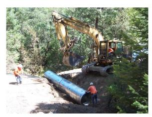
**Upper Left**: Installing a new culvert with armored outboard fill on Indian Creek Road (2008) **Upper Right**: Installing a 42" pipe in a Class III stream crossing on Deerlick Springs Road (2009)
