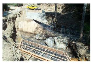
Whites Gulch (Siskiyou County) outlet jump (**upper left**) in October 2008 and new abutment form work in August 2009 (**upper right**). The last segments of the culvert were removed on September 23<sup>rd</sup> and the bridge is now open for travel (**lower left view from outlet area**). Seeding and mulching of the old road approaches was completed on October 15 (**lower right**) and tree planting is scheduled for winter 2009.
