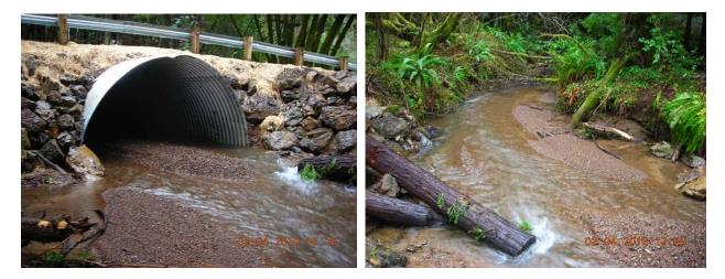
Below: The 16' wide culvert on White's Gulch with outlet jump compared with the new bridge in fall 2009.
