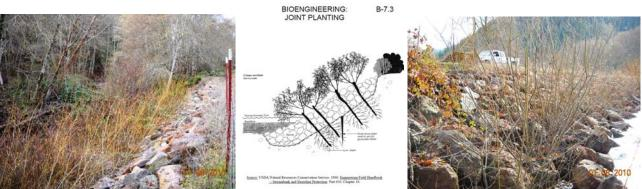
Above: Bar Road Storm Repair (Siskiyou County) repairs made in 2008 (after the 2006 storm damage) included implementing joint planting within rock slope protection. Photos taken January 2010.
