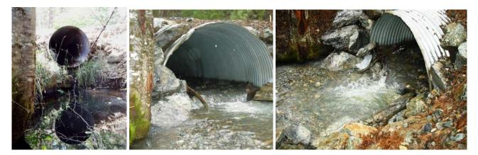
Above Left: Finley Gulch was a 42" diameter culvert with a 2' jump at the outlet. It was replaced with an 84" embedded culvert (center and right photos) and designed with a 5" jump into the outlet.
