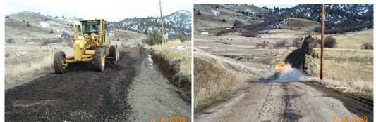
All five counties use asphalt grindings to surface unpaved roads or resurface chip-sealed roads. The photos above demonstrate placement of grindings on York Road (Siskiyou County).
