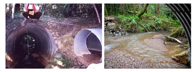
The Ancestor Creek crossing consisted of a 7' and 3' diameter culvert (left). These pipes were replaced with a 16' wide, embedded multiplate arch culvert (above right and below). Installing culverts utilizing the active channel design can allow for natural stream function and large wood placement, as depicted below.
